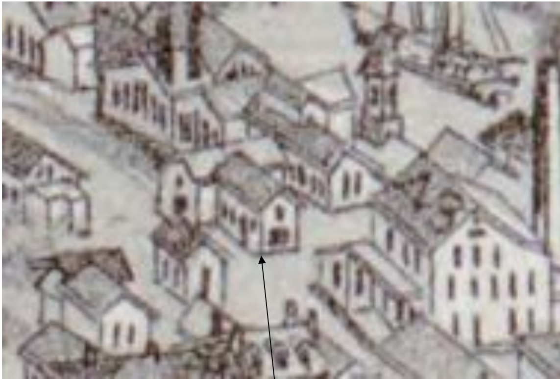
Cumberland Nail and Iron Company Office
